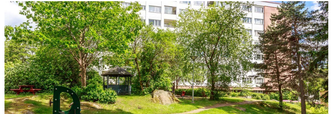
Eriksberg 17:1: Refurbishment of properties for public use, total amount SEK 186 million and invested so far SEK 128 million. Planned completion Q2 2018.
